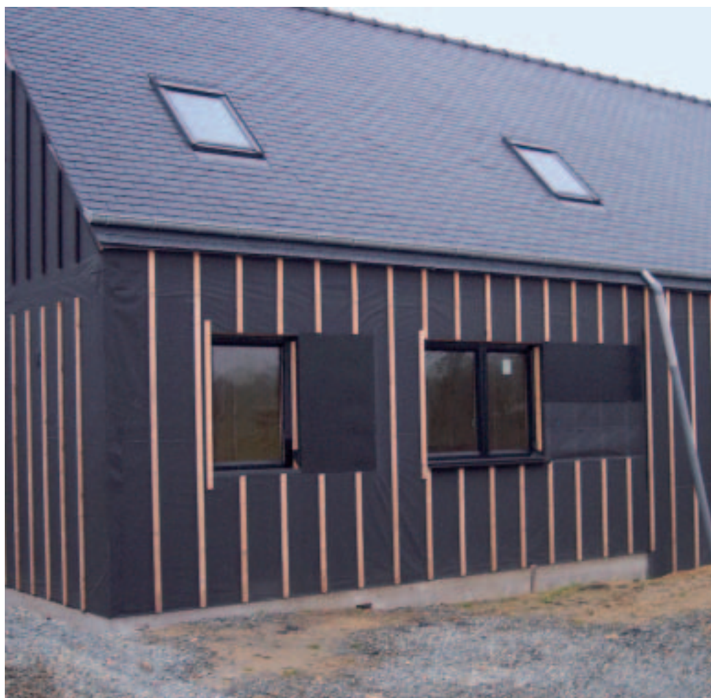
DELTA®-FASSADE S offers safe protection under open facings with joints up to 50 mm wide.
