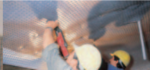
In tunnels, DELTA®-PT supports shotcrete applications.
