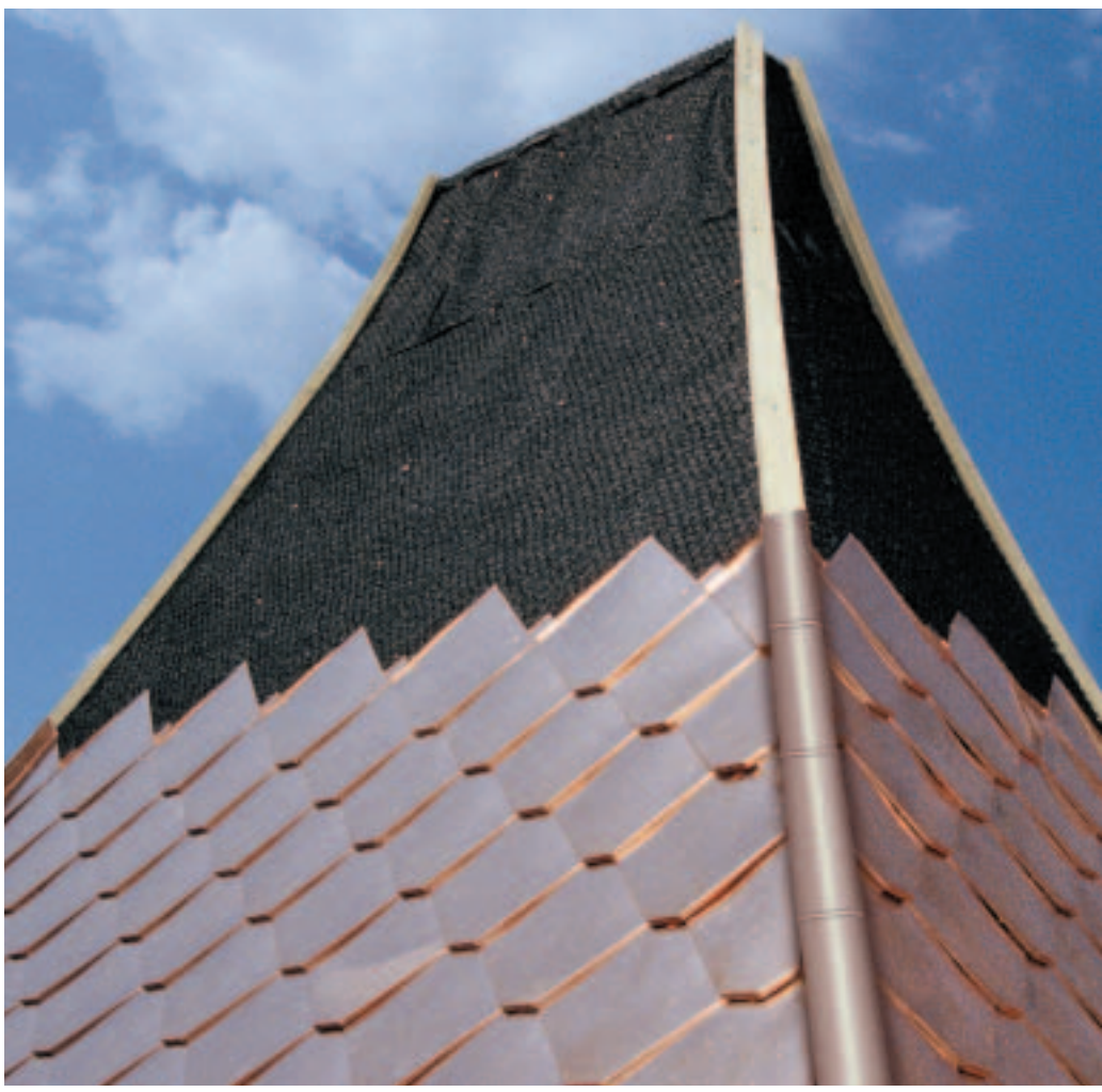
DELTA®-TRELA is the optimum air-gap sheet for high-quality metal roofs.
