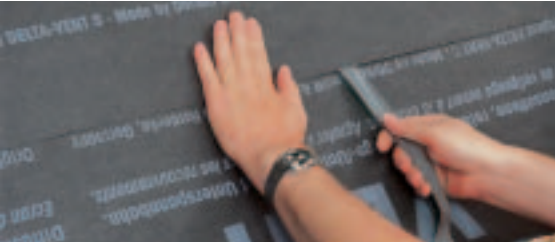
Wind-tight overlap seams with DELTA®-VENT S PLUS.
